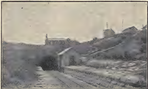
FIG. 67—Grand Trunk Railway Tunnel under the St. Clair River, Sarnia, Ont
